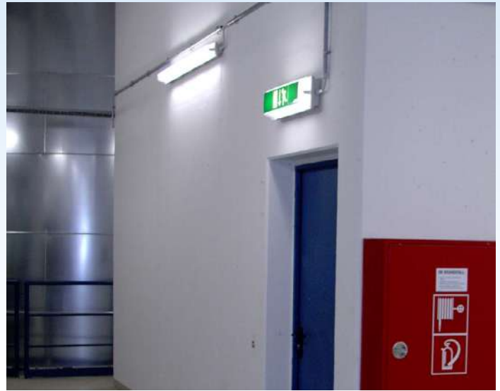
Integration of self-contained emergency luminaires - Emergency luminaires can be used with the following three types of circuit: Continuous light, standby light and controlled light.
